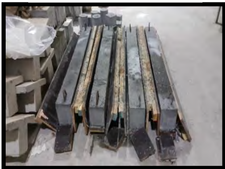
(e) Removal of formwork
