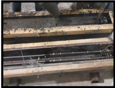
(d) Beams during concrete casting
