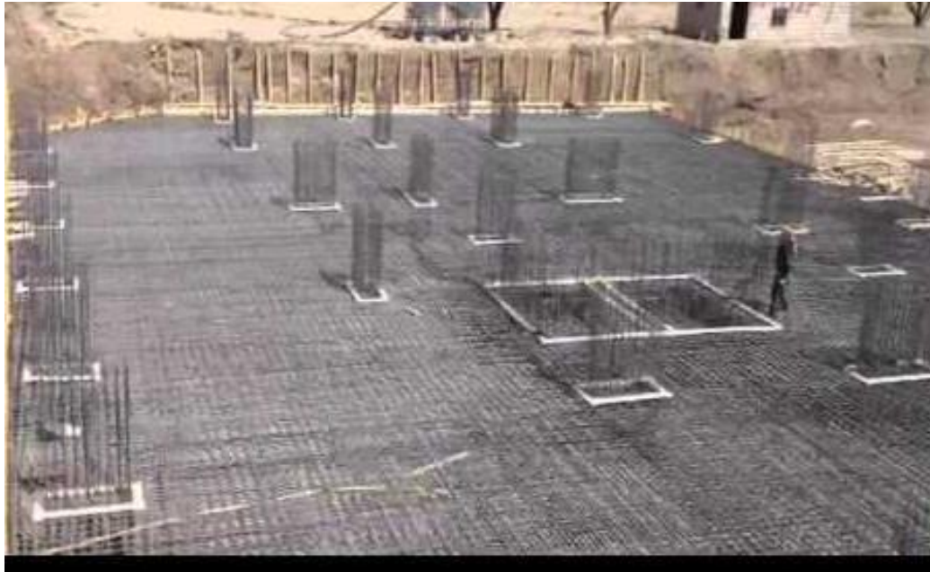
Figure 7: Example Mat Foundation [5]
