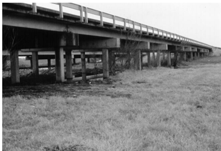
Figure 24: Big Creek Relief bridge [44]
