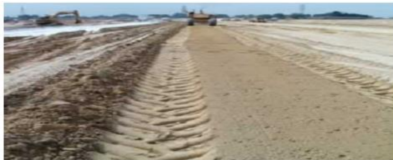
Figure 2-11: Final Mixing and Pulverization [48]
