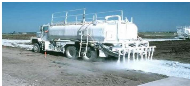
Figure 2-9: Lime Spreading [48]
