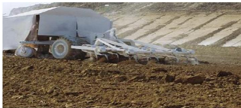
Figure 2-8: Scarification and initial pulverization of Soil [48]
