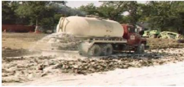
Figure 2-10: Preliminary Mixing and Watering [48]
