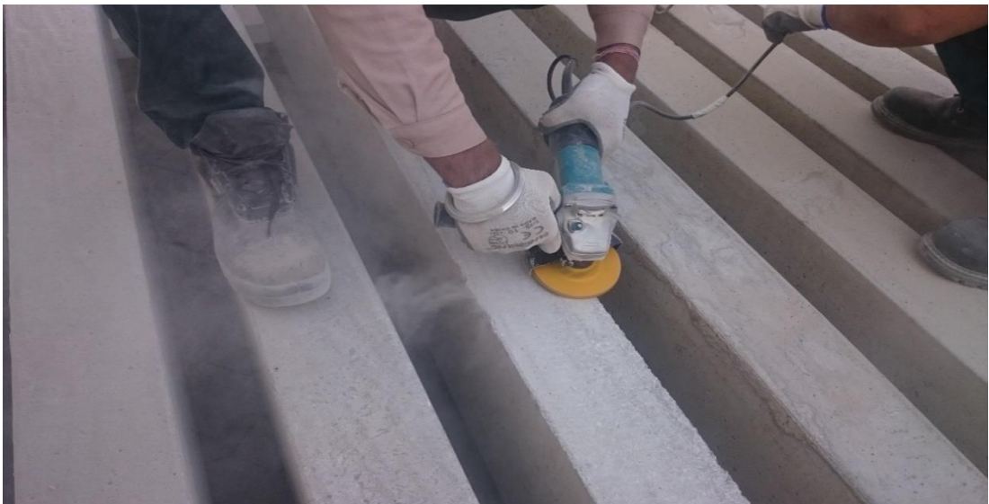
Figure 25: Surface grinding of RC beams
