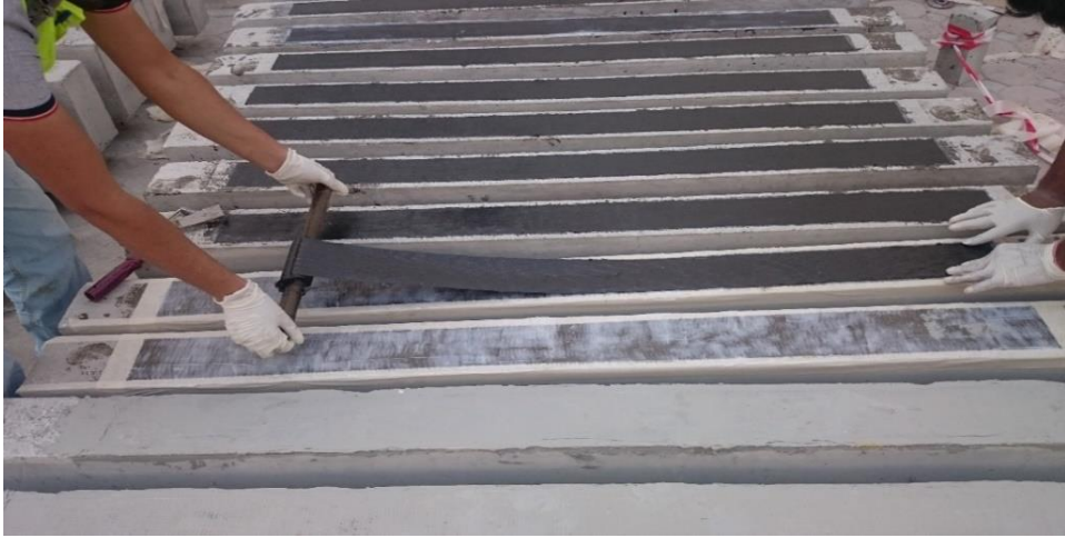
Figure 28: CFRP installation
