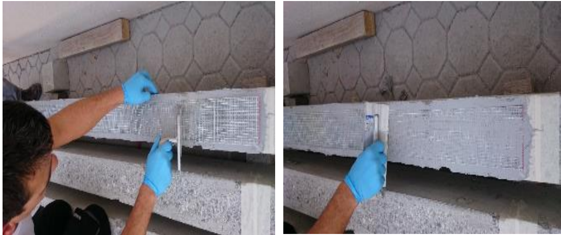
Figure 26: SMM installation
