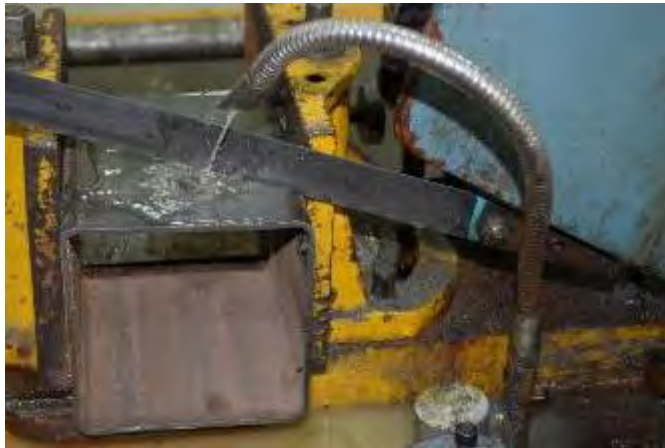
Figure 33: Cutting ISSSBs from hollow structural steel
