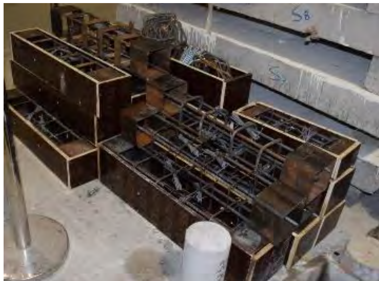
Figure 37: Placement of steel cages in formwork
