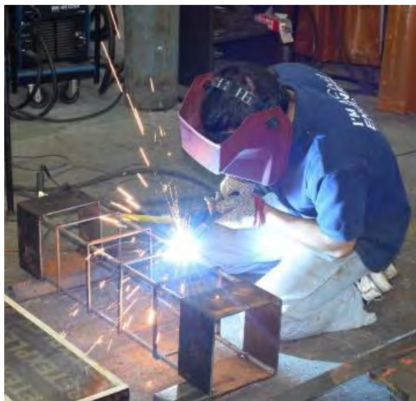
Figure 34: Assembling and tack-welding the steel cage
