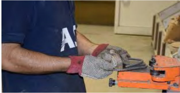
Figure 32: Making end hooks on ties using the steel bender
