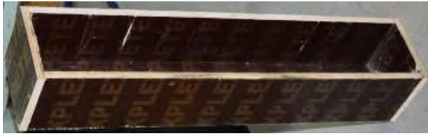
Figure 31: Example of completed wood formwork
