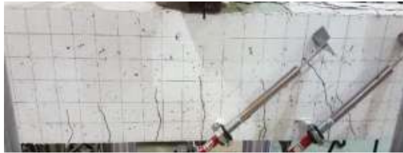
(c) Post-cracking stage
