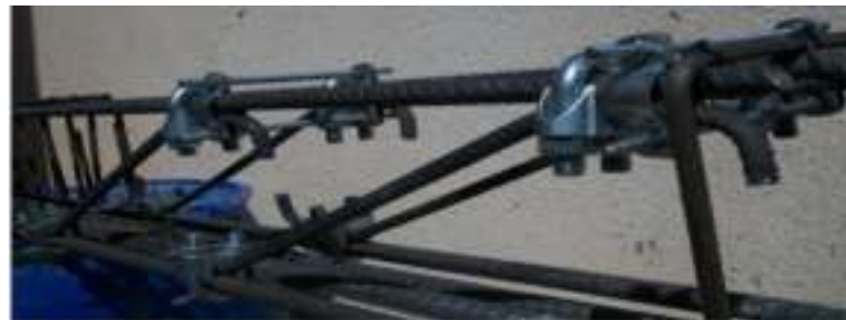
(a) Bolted swimmer bars using threaded bar.
