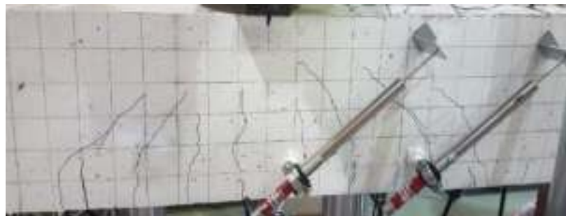
(c) Post-cracking stage
