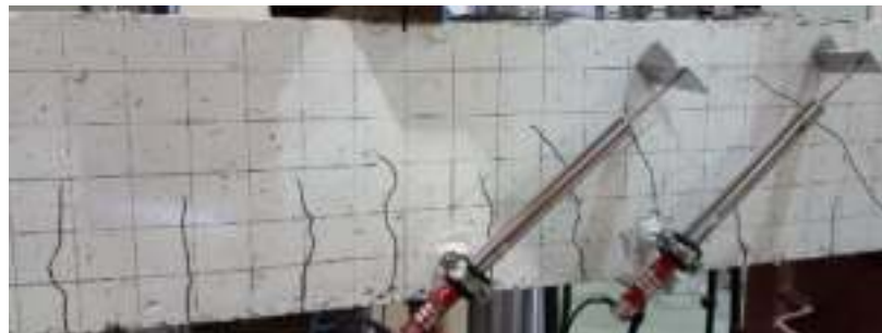
(c) Post-cracking stage
