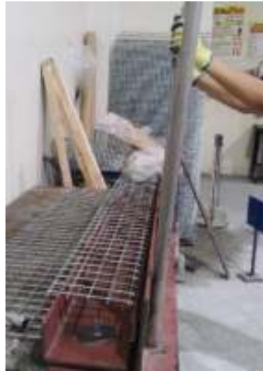
Figure 76: Preparing WWF steel cages using bending bench.
