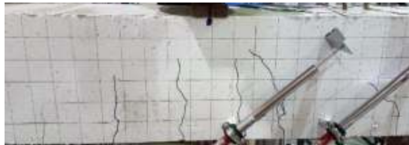
(c) Post-cracking stage
