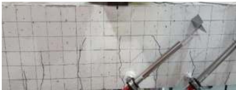
(c) Post-cracking stage
