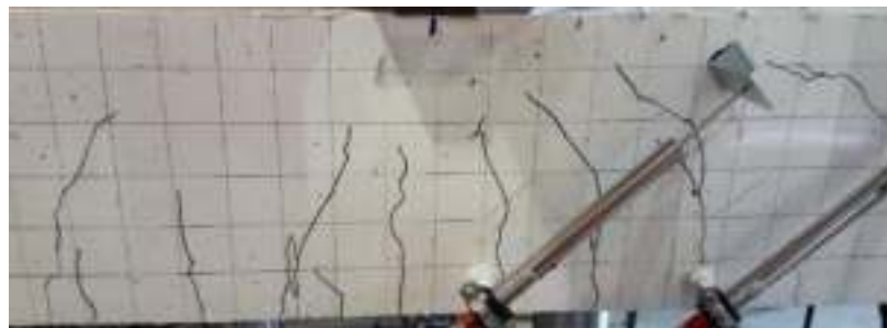
(c) Post-cracking stage
