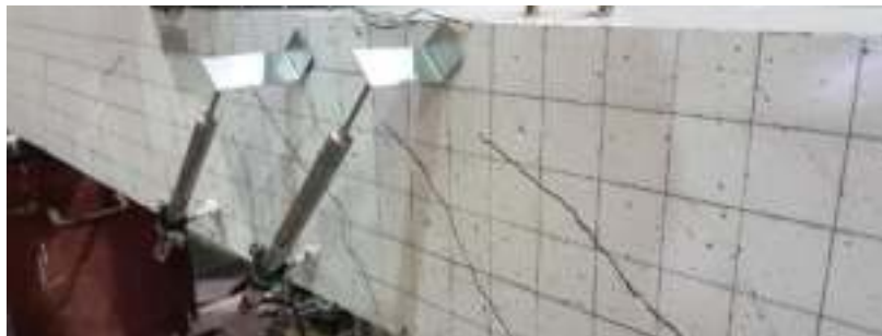
(c) Post-cracking stage
