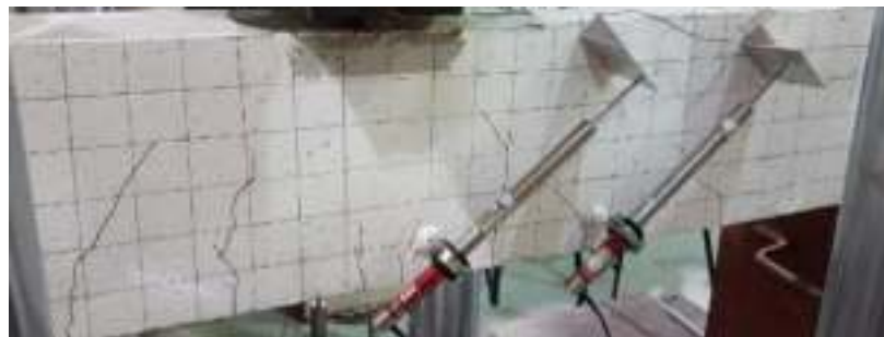
(c) Post-cracking stage
