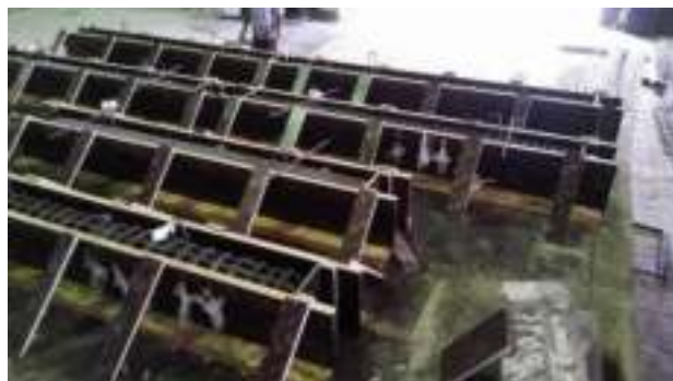
Figure 78: Formwork prepared on top of the vibrating bench.
