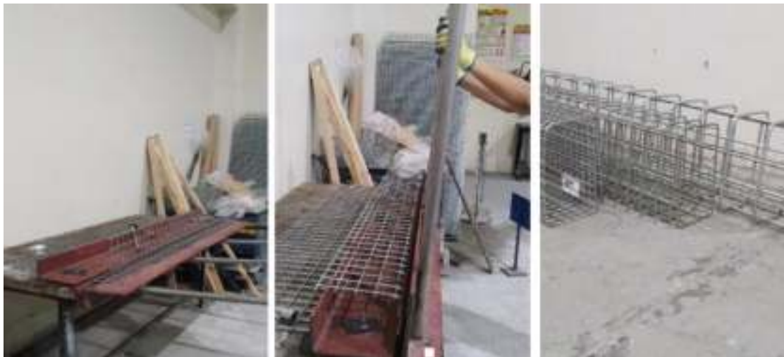
Figure 75: Preparing the WWF cages using the new method.
