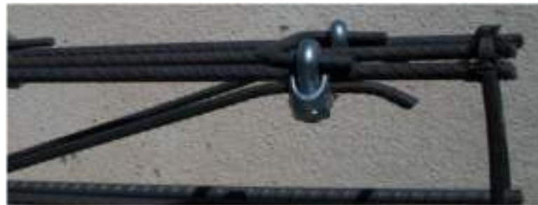
(b) Bolted swimmer bars using U-link.
