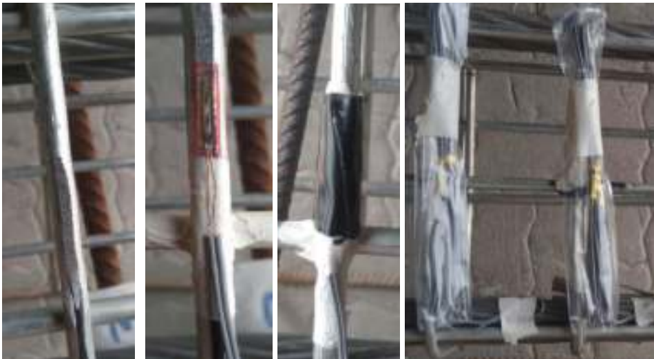
Figure 77: Attaching strain gauges to steel cages.
