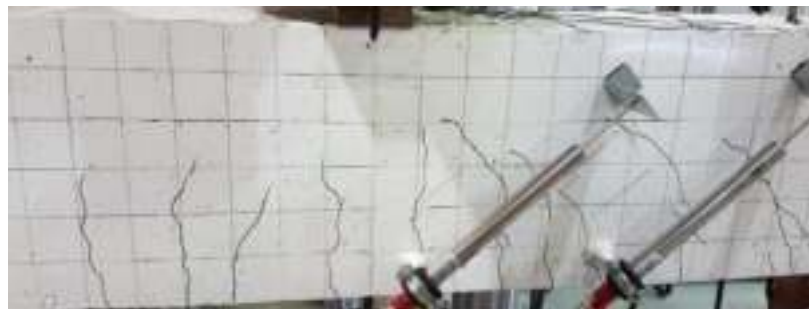
(c) Post-cracking stage
