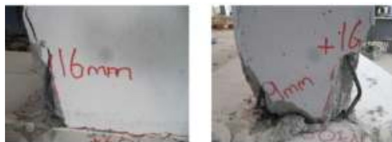
Figure 32: Buckling of vertical wires of WWF cage [33].
