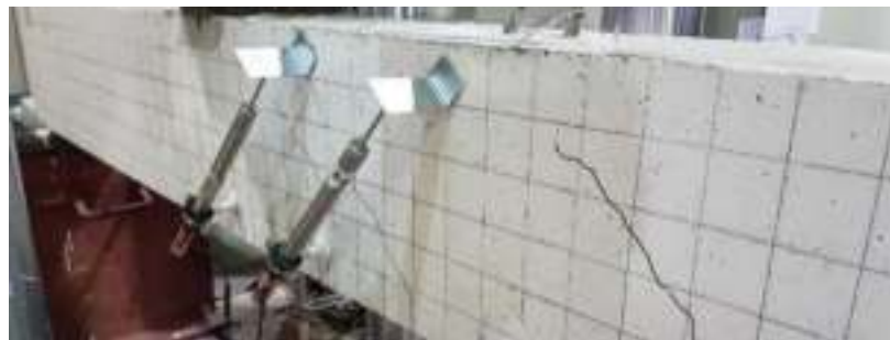
(c) Post-cracking stage
