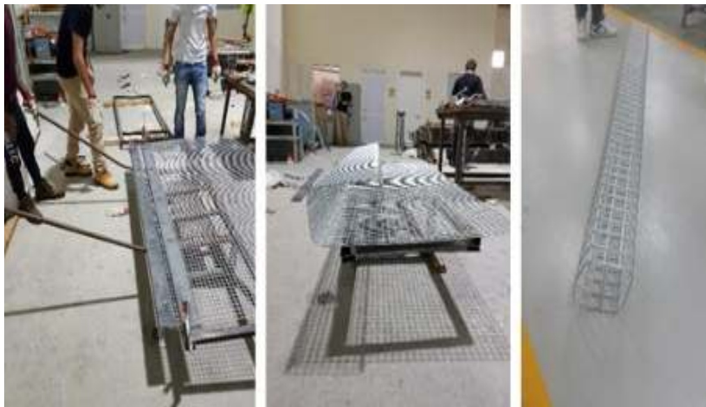
Figure 71: Preparing the WWF cages using the old method.
