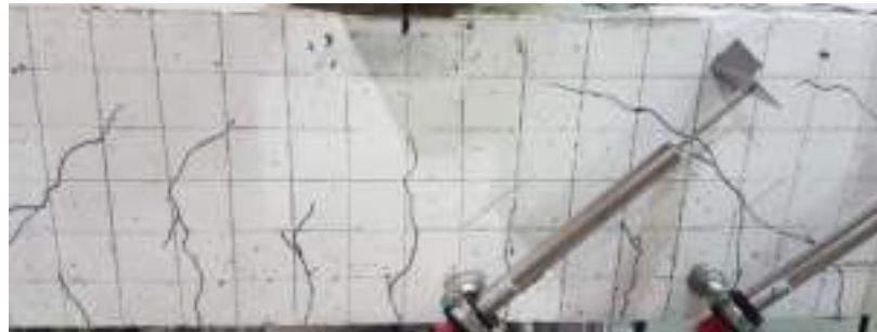
(c) Post-cracking stage
