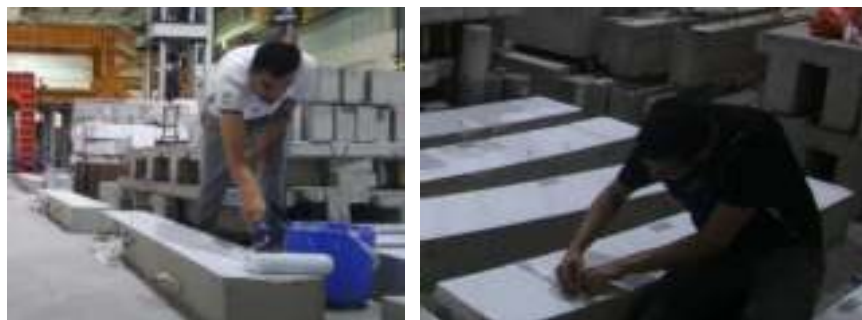
Figure 81: Painting and constructing gridlines process.
