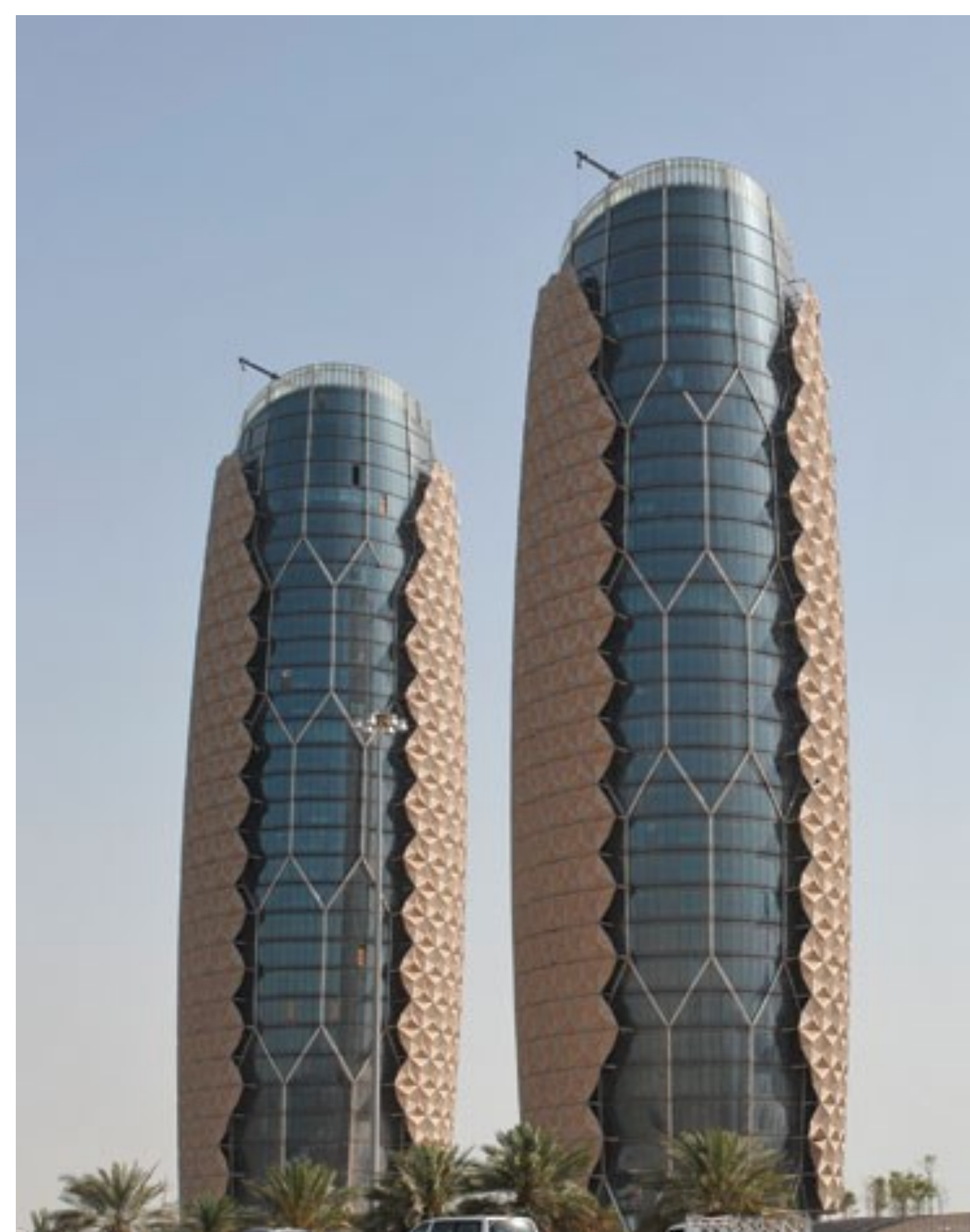
Figure 1: Similar existing project (Al Bahar Towers)
