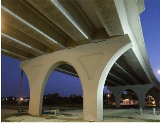
(a) Concrete girders
