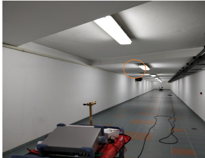
Figure 3.7: The Underground Tunnel.
