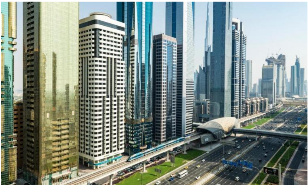
Figure 4.1: Image of one of the streets in Dubai (UAE) and the common constructions style in Dubai.
